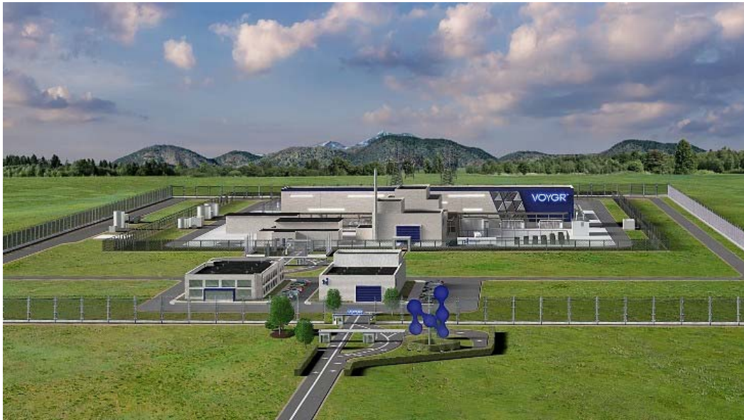
Image: NuScale VOYGR SMR, 6 x 77 MWe modules, 462 MWe total on 13 hectare site.
